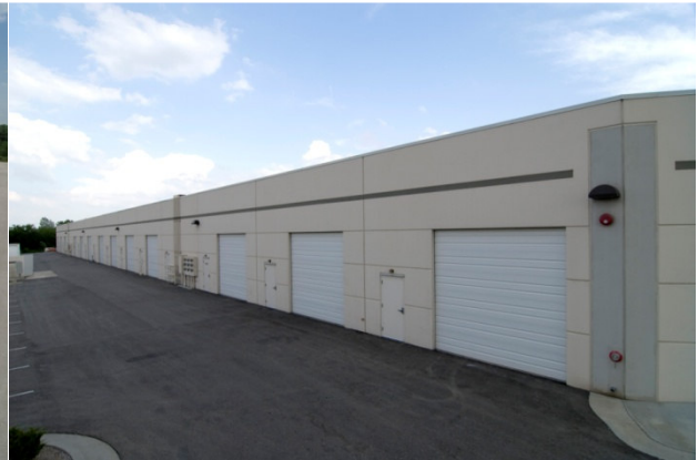
(DRIVE IN DOORS ALLOW EASY ACCESS )
